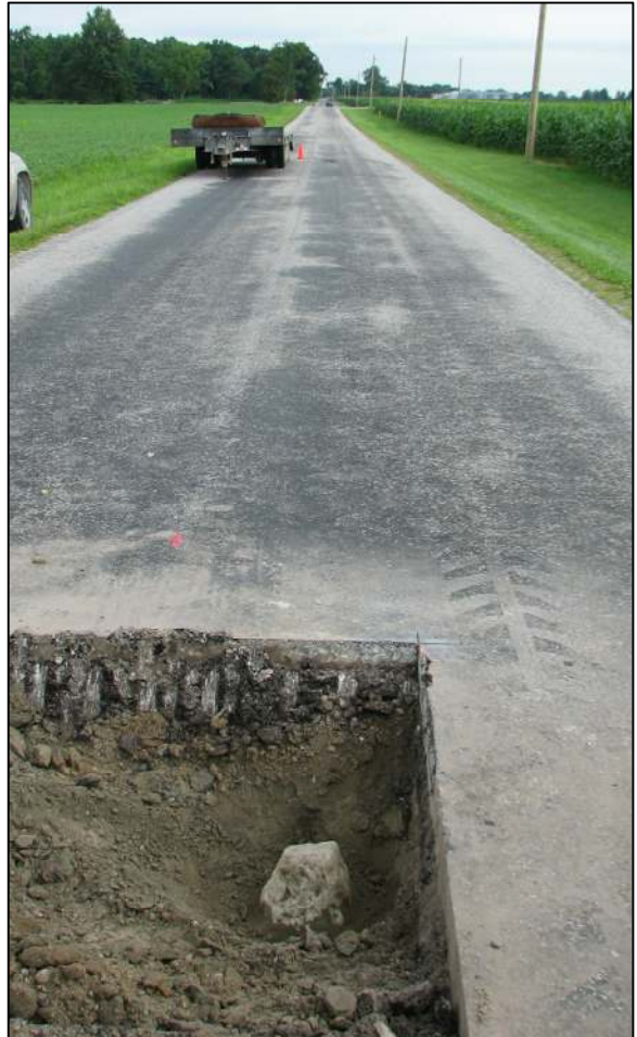
View from the south, looking across the stone and north along County Road 500 East.
