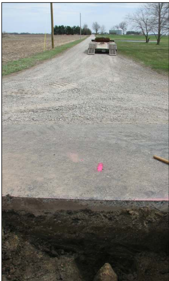
View from the west looking across the stone (in shadows) and east along County Road 400 North.
