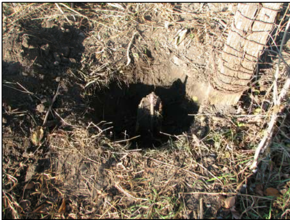
The standing post and the base of the old post, with rebar, from above and east.
