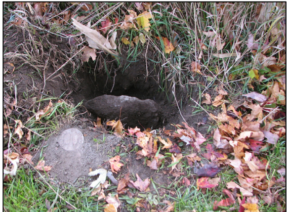
The stone at the standard corner, and the harrison monument found. See documentation.
