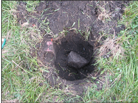
View from above showing the stone at the closing corner and the railroad rail.
