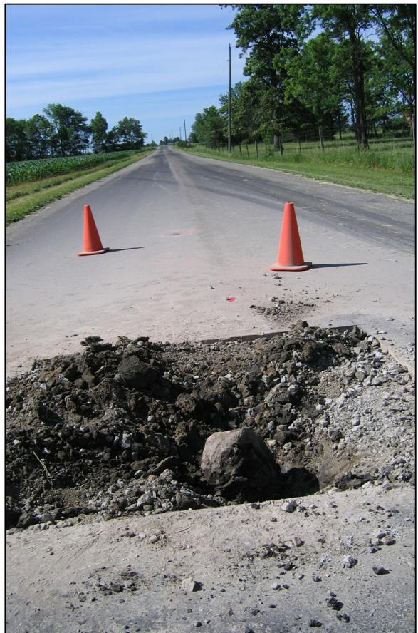
View from the north, looking across the stone at corner 2 and south along County Road 600 East. The stone is shown stood up in a vertical orientation in this picture. Corner 1, not yet excavated, is visible in the foreground.
