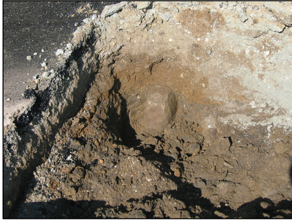
View of the stone as first exposed.
