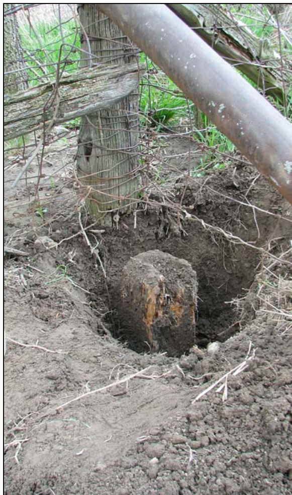
Base of old cedar post exposed. View from northwest.
