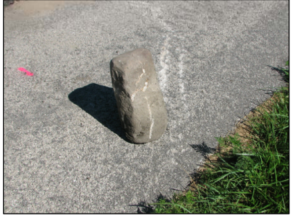
The stone, removed from the road.
