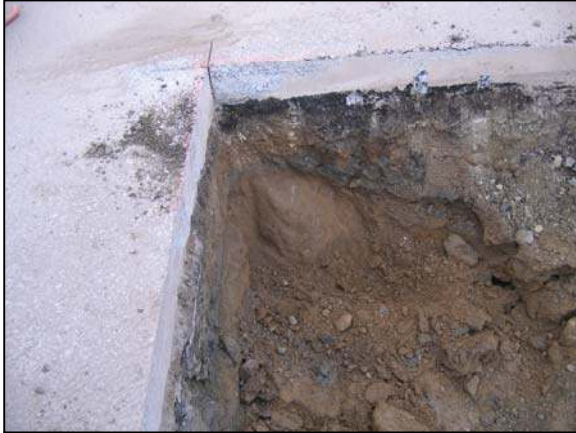
Corner stone. View of east side of stone as intially exposed.
