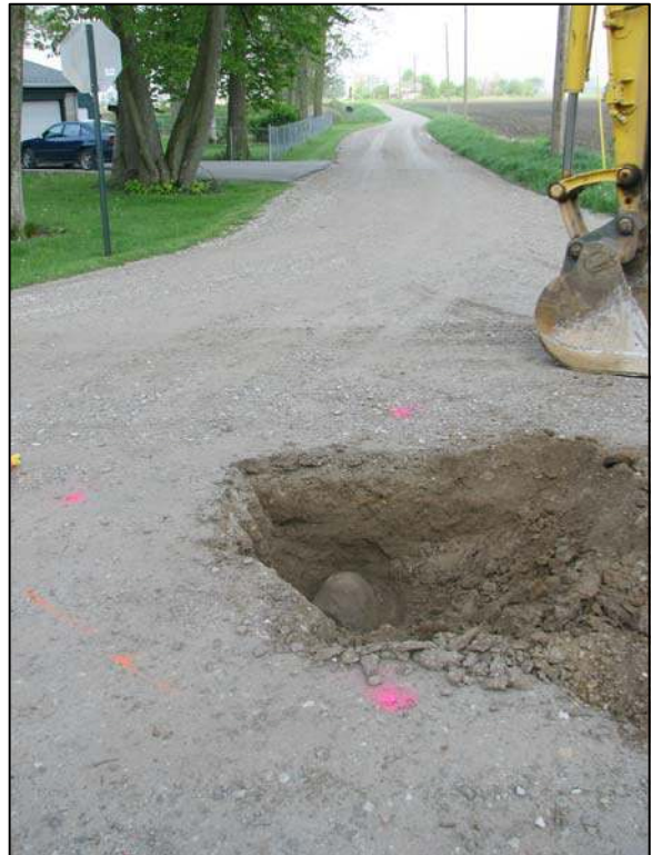
View from the east looking across the hole and along County Road 500 South to the west.
