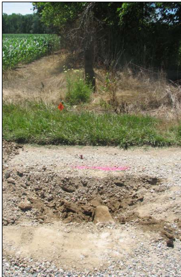
View looking across the stone to the wood end post on the south side of C.R. 700 North.
