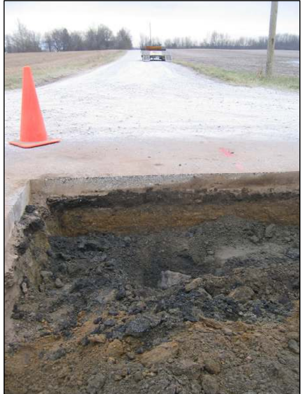
View of the stone and County Road 700 East, from the north, looking south.
