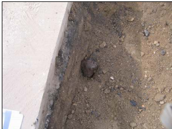
View of the piece of wood above the stone.
