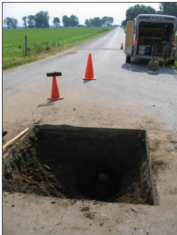
View of the from the west, looking across the stone in shadows, along C.R. 100 North. Note the piece of wood visible on the safety cone.
