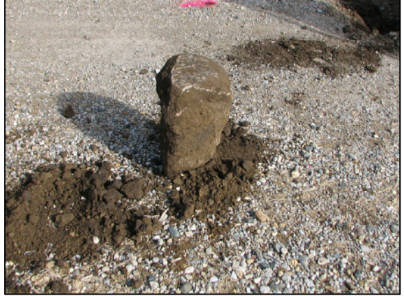
The stone removed from the road bed.
