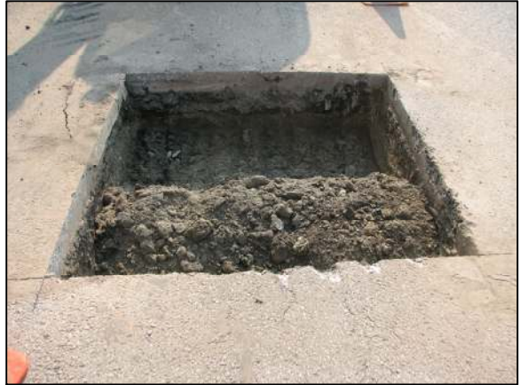
The area of excavation at the closing corner.
