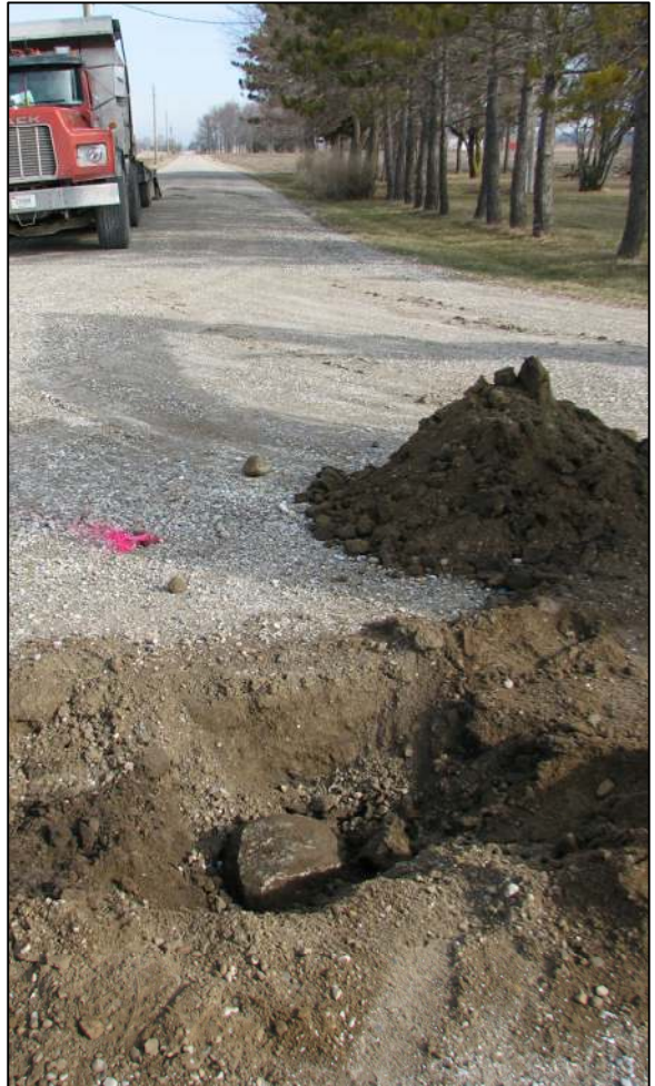
View from the south, looking across the stone and north along County Road 100 East.
