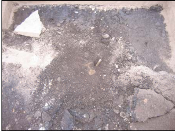
Railroad rail and rebar, as found.
