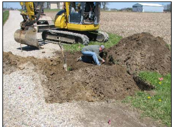
View from the south, showing the area of excavation. Brandon Miller, Miller Excavating, is inspecting the upper stone as found.
