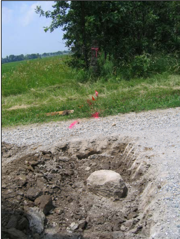
View from the east, showing the stone and the post on the west side of the road.
