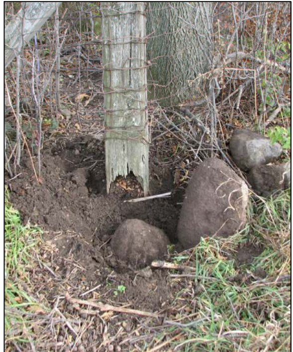
Several rocks excavated from around the post.
