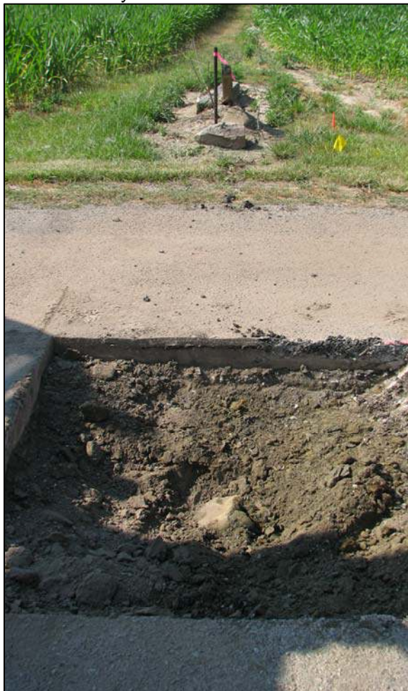
View of the stone and the posts on the south side of County Road 400 South.
