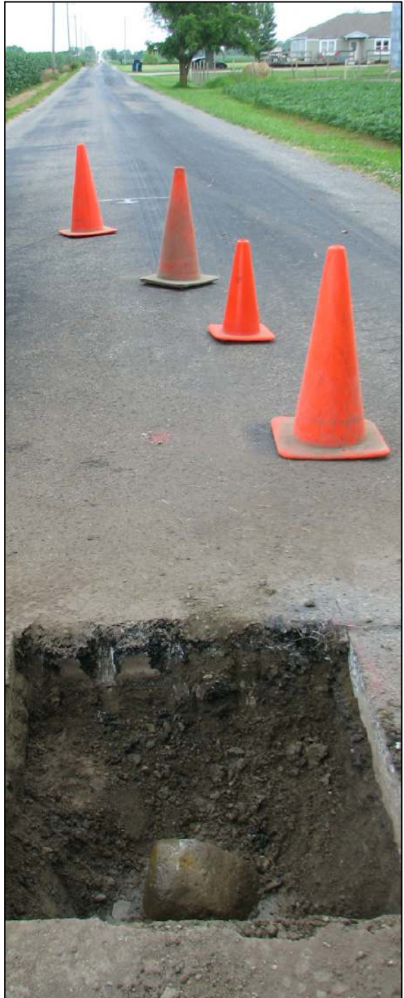
View from the south, looking across the stone and north along County Road 900 East.
