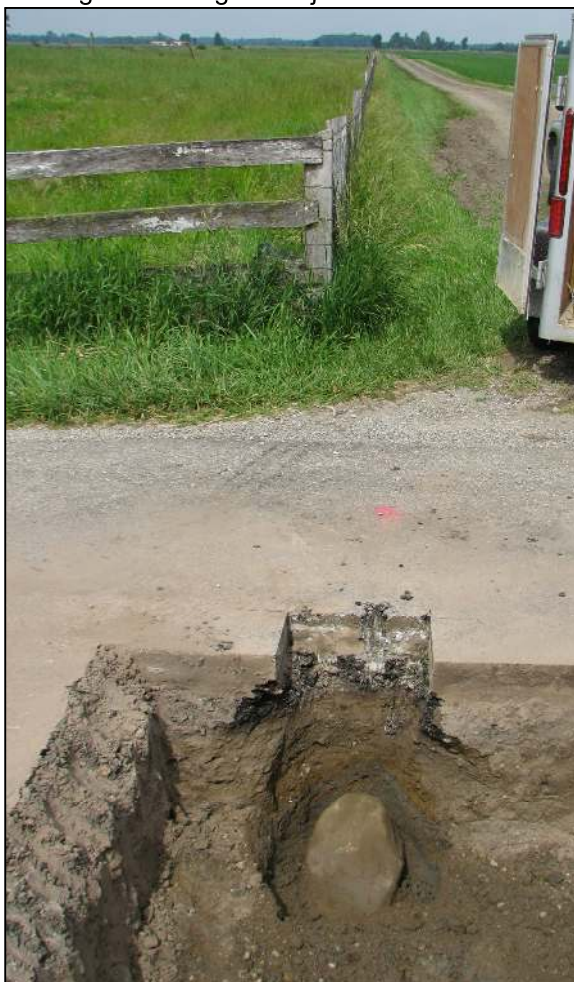
View from the east, looking west along the adjacent fence line.
