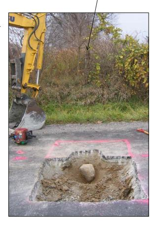
View from above and slightly south of west. Clay sub-base has been excavated from around the stone almost to the bottom of the stone.
