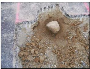
View from above and west. Hole and indention in the clay sub-base after the stone was removed. Harrison monument was set in the position of the midpoint of the top of the stone.
