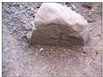
Photograph taken from Northeast, showing area of excavation as it is being re-filled with gravel. The main hole is 4 feet by 4 feet centered on the railroad rail (see notes, other sheet). Record stone was found in bottom of the offset square in the S.W. corner of the main hole. The small witness stone found above the record stone is shown along with several small rocks on pavement at the top right corner of the photograph.
