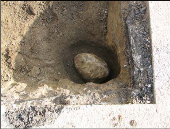
Corner stone - overhead view from south.
