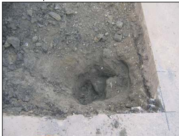
The south top stone (right) and the lower stone as first exposed.
