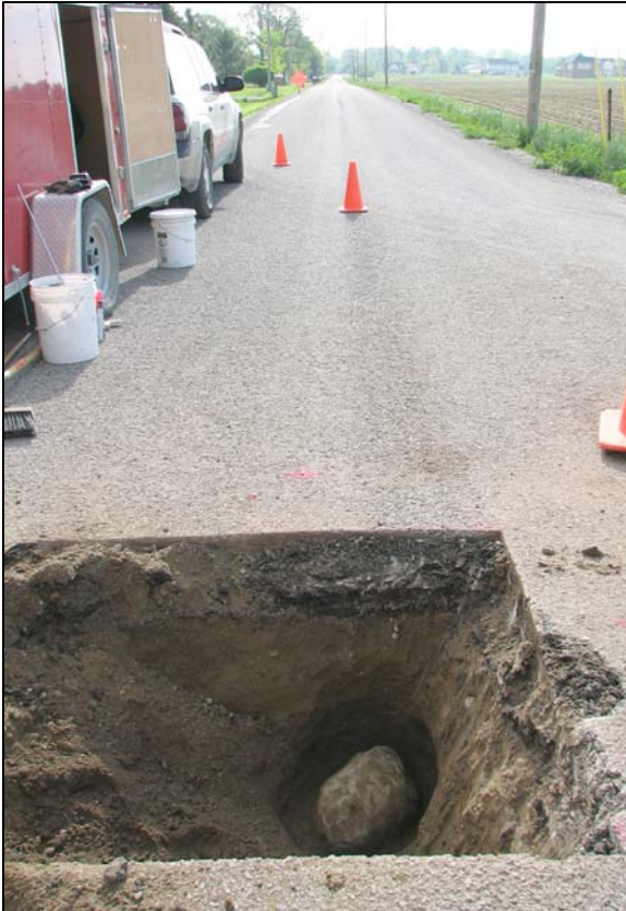
View from west, looking across corner stone and along County Road 400 South to the east.
