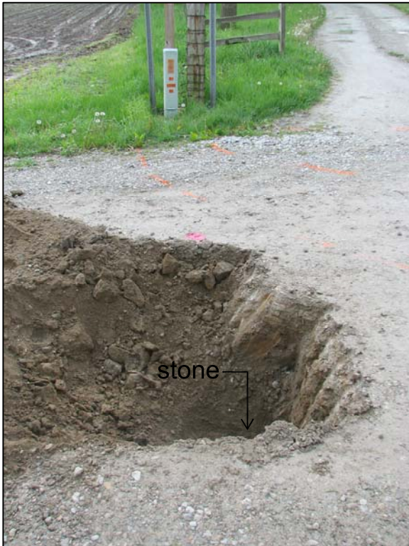
View from west, looking across hole to wood end post at the terminus of an old fence to the east. The stone is not visible, but shown by arrow.
