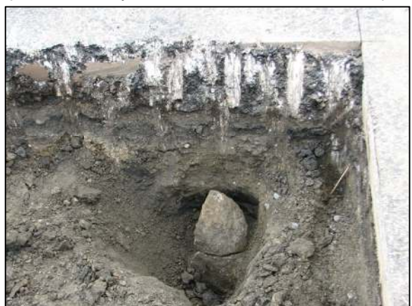
Both parts of the stone. The top part has been placed directly on the still embedded bottom part.
