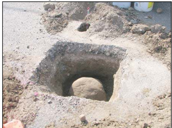
Corner stone and railroad rail from north. The chaining pin is on the rail.
