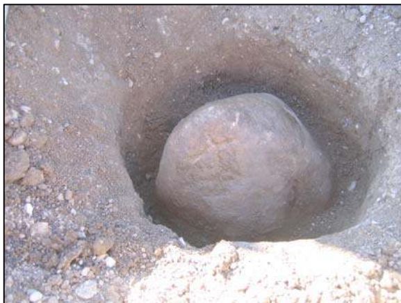
Corner stone - overhead view from the north. The "+" is on the north side of the stone, approximately 3" down from the top of the stone.
