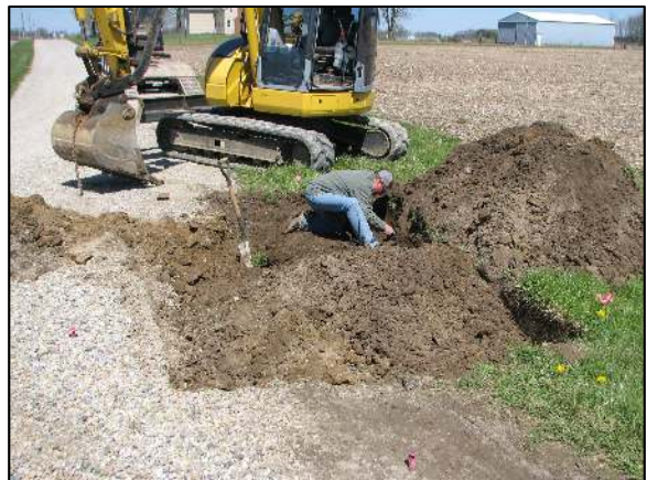
View from the south, showing the area of excavation. Brandon Miller, Miller Excavating, is inspecting the upper stone as found.
