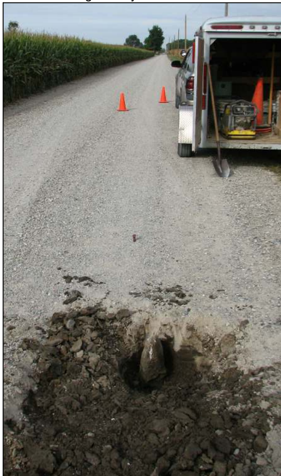
View from the east, looking across the stone and east along County Road 700 North.
