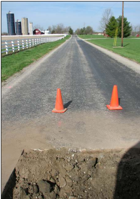
View from above the stone, looking west along County Road 200 North.
