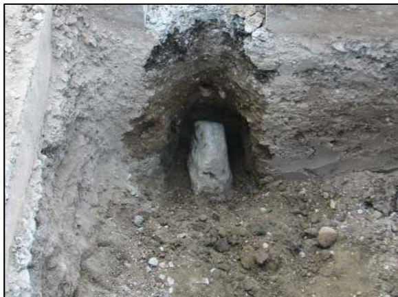
The stone at Corner 2 (Hamilton County corner) fully exposed.
