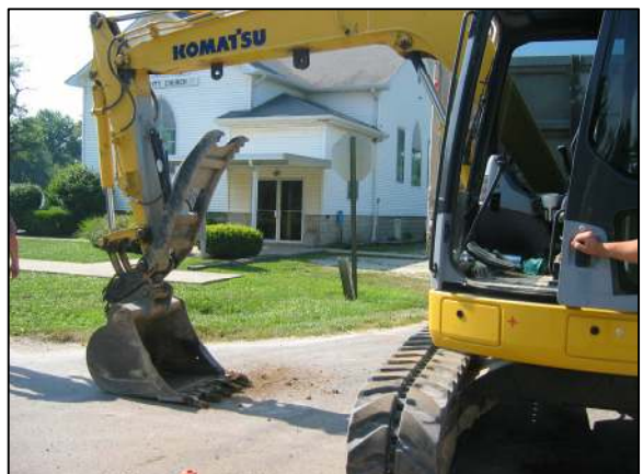
Big Springs Community Church, from above the stone at the time of excavation.
