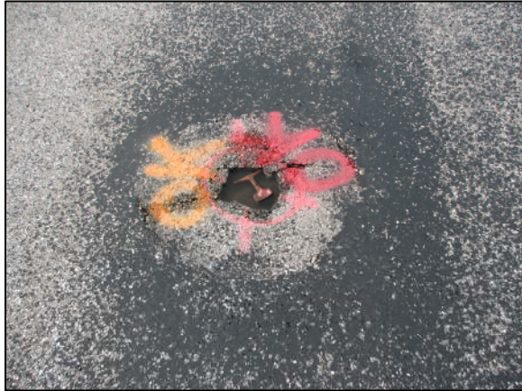
The top of the rail prior to excavation.
