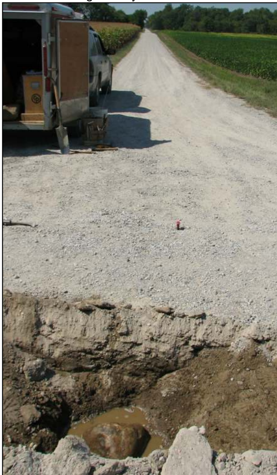
View from the east, looking across the stone and west along County Road 900 North.
