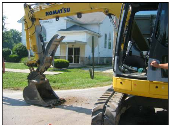
Big Springs Community Church, from above the stone at the time of excavation.
