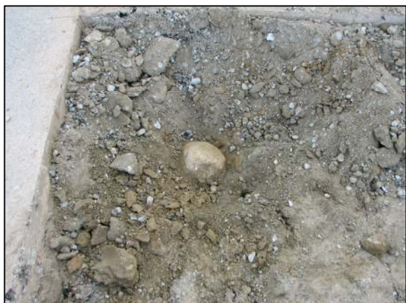
The stone at corner 1.
