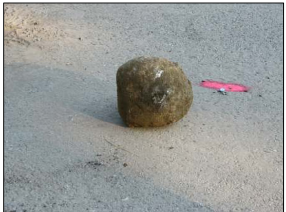
The stone as removed from the road bed.
