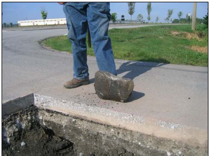
The stone removed from the road bed and situated in the orientation at which it was found.
