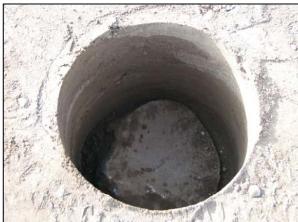
The lower stone immediately before it is encased in concrete and a harrison monument set over it.
