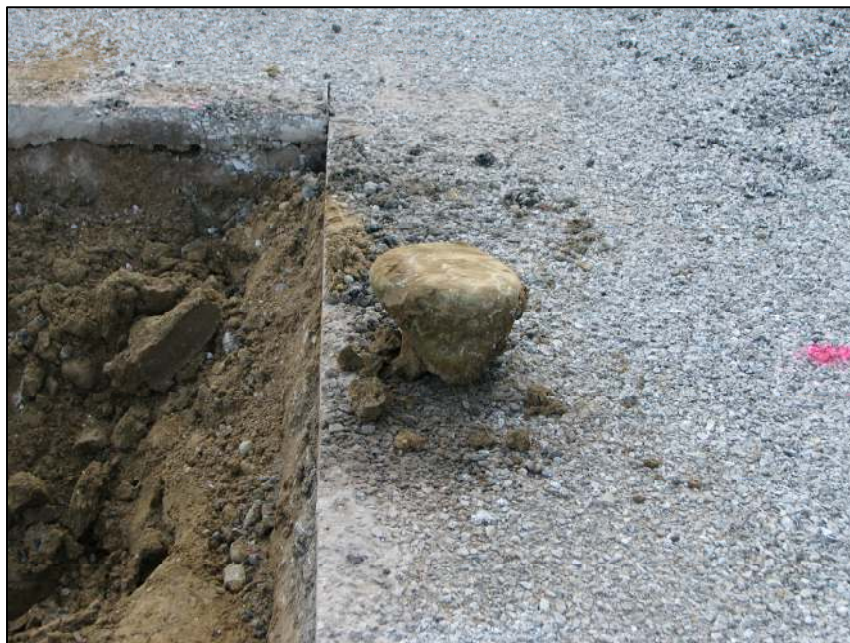
The stone removed from the road.
