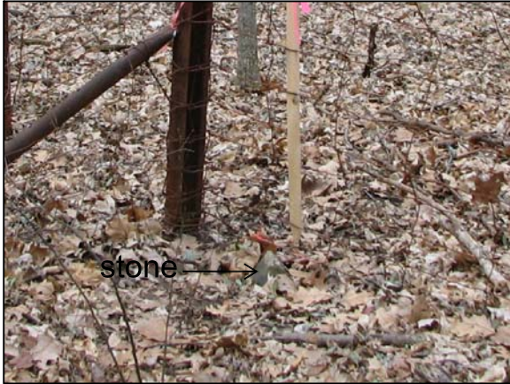
Corner stone as visible prior to excavation - view from southeast.
