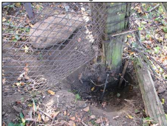
The post and iron pipe. The small rebar is in the position at which the harrison was subsequently set. The stone is on the ground to the left.
