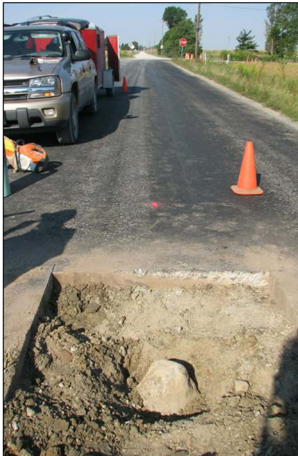
View from the east, looking across the stone and west along County Road 100 North, across U.S. 421
