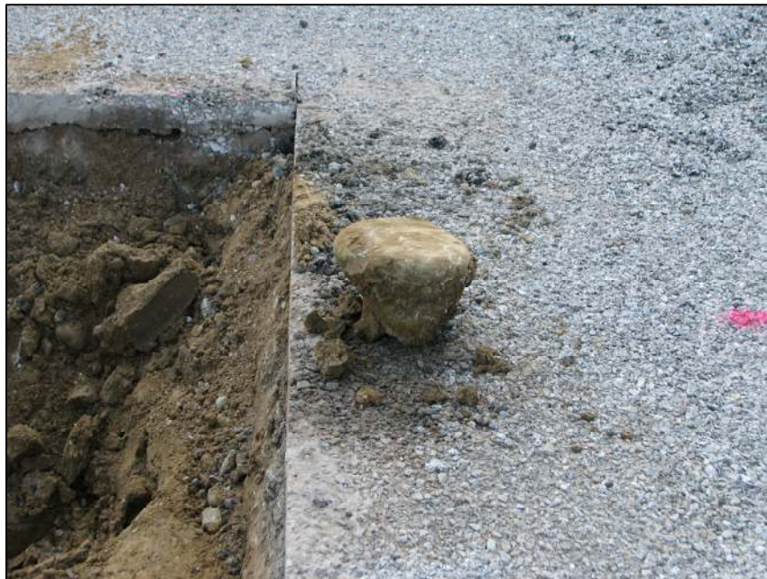
The stone removed from the road.
