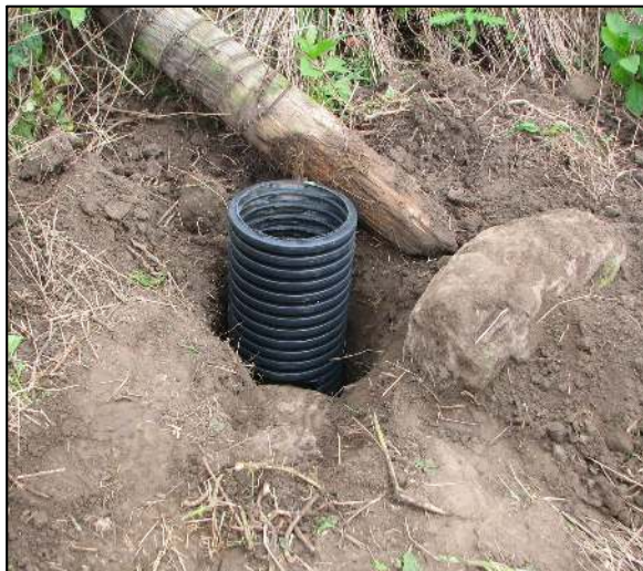
A vertical section of storm pipe, to be filled with concrete to support the Harrison monument.
