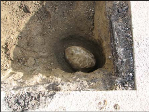
Corner stone - overhead view from south.
