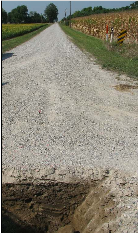
View from the east, looking across the stone and west along County Road 900 North.
