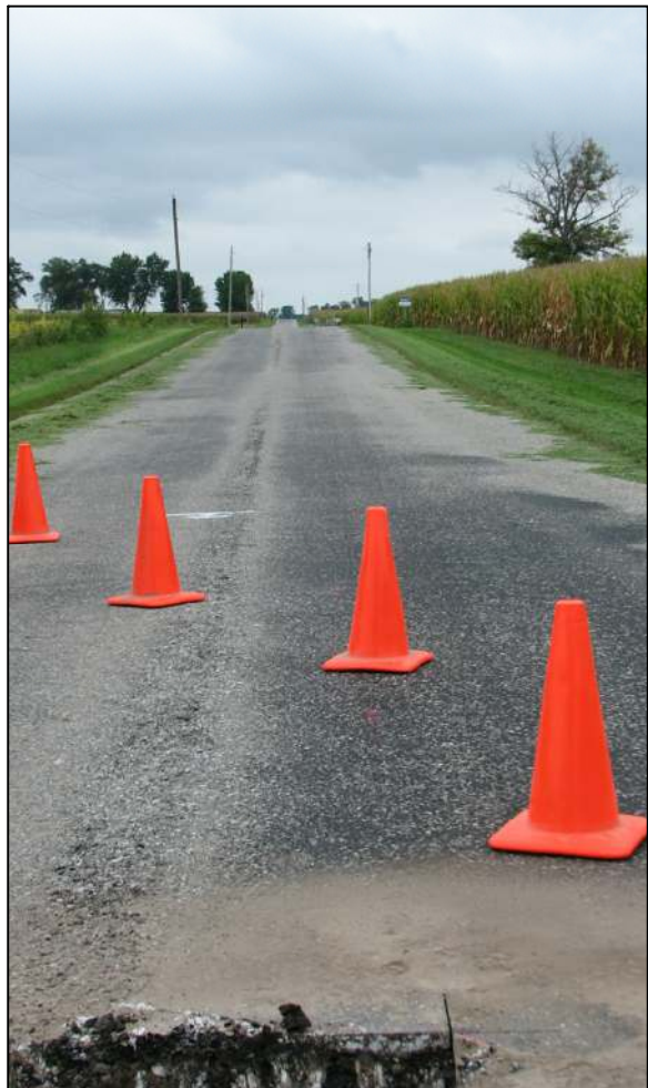
View from above the stone, looking north along County Road 400 West.
