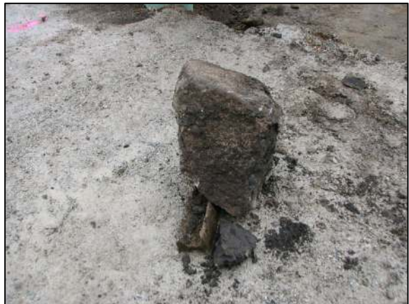
The stone (supported by the rail) after removal from the road bed.
