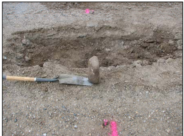
The stone removed from the road.
