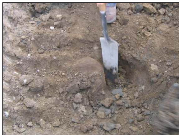
The stone being exposed. Further pictures are not available due to camera failure during excavation.
