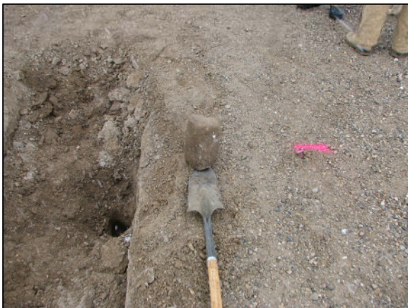
The stone removed from the road.
