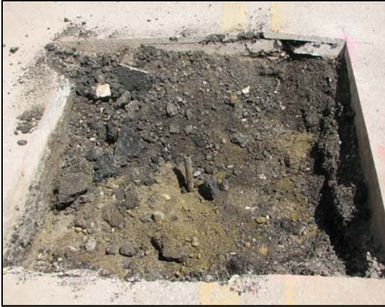
Iron pipe, into which rebar was driven.
