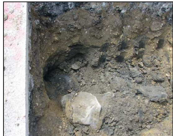
Thin stone shifted to side, revealing top of record corner stone.
