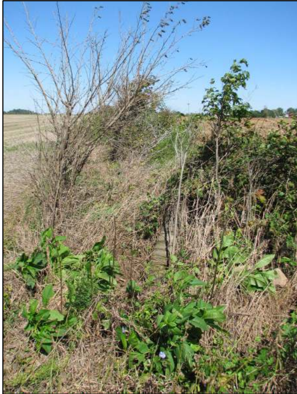
The corner prior to excavation. View of the leaning corner post from the south.
