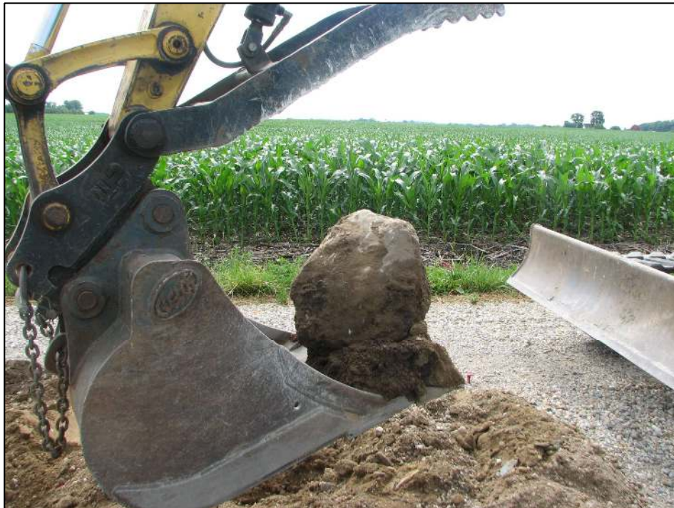
The stone as it is being removed from the road bed.
