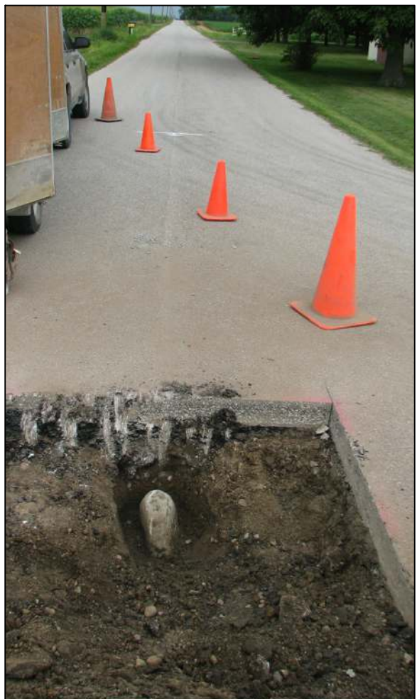
View from the east, looking across the stone and west along County Road 850 North.
