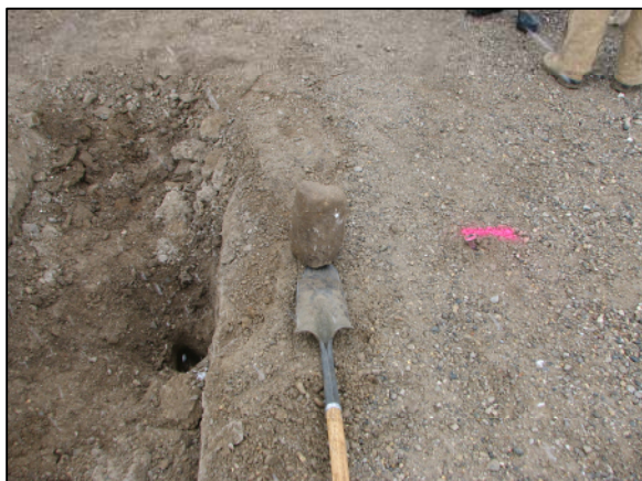
The stone removed from the road.
