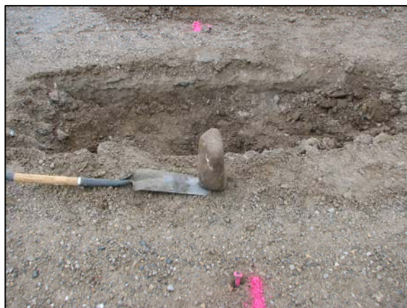
The stone removed from the road.
