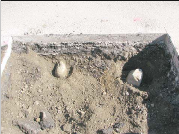
Lower record corner stone (left) and witness stone to east (right)
