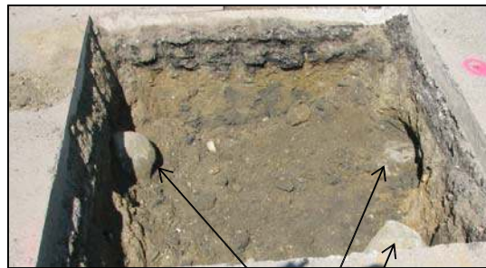
witness stone to south lower record corner stone witness stone to east
