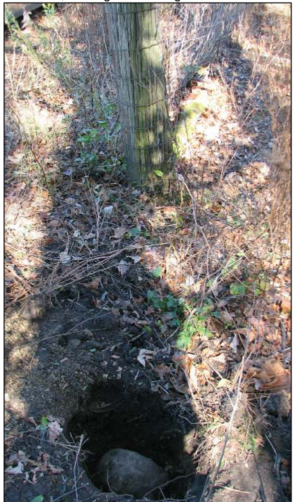
The stone and the wood end post. View from the south, looking north along the N-S fence.
