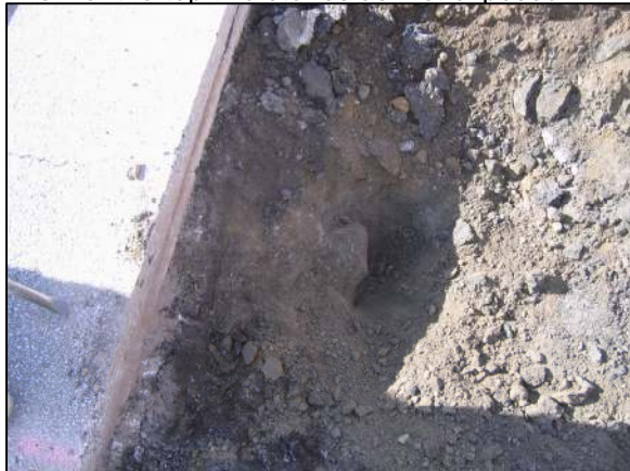
View of the top two stones as first exposed.
