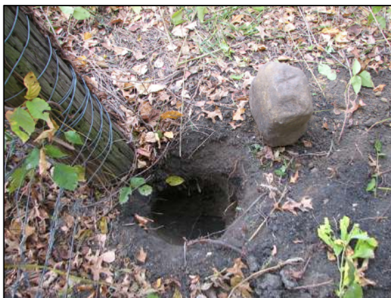
Same as above, view from opposite direction.
