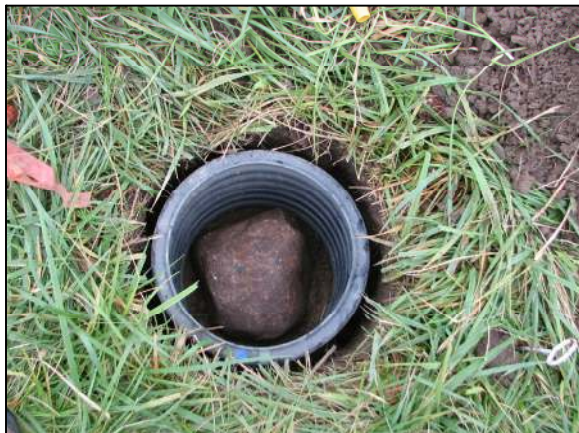
The stone at corner one prior to being encased in concrete with a Harrison monument set above.
