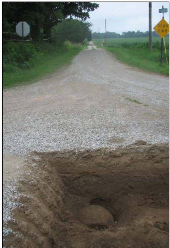
View from east, looking across the stone and west along C.R. 950 North to the west.
