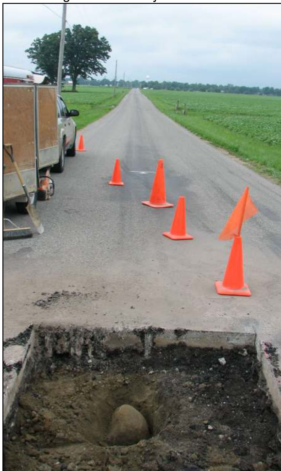
View from south, looking across the stone and north along Clinton County Road 850 West.
