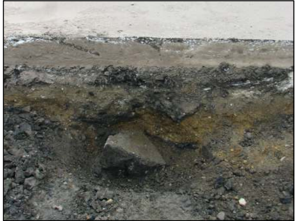
The more fully exposed, viewed from the west.
