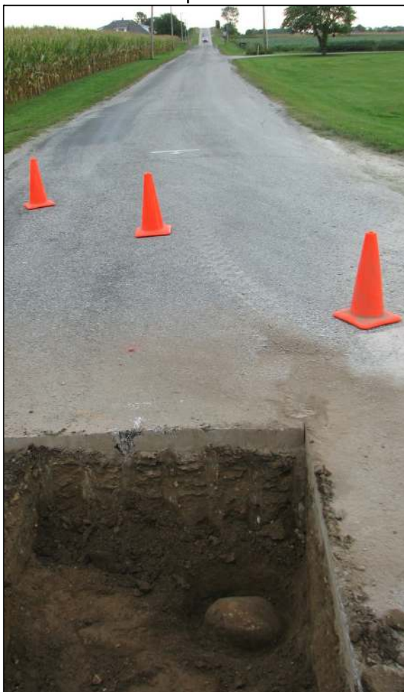
View from the west, looking across the stone and east along County Road 950 North toward the Interstate 65 overpass.
